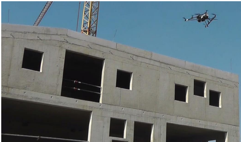
Fig. 4. Octocopter with Nex-7 camera mounted in front of the construction site.
