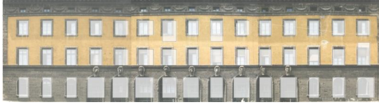
Figure 10: Example for the reconstruction result of a single façade.
