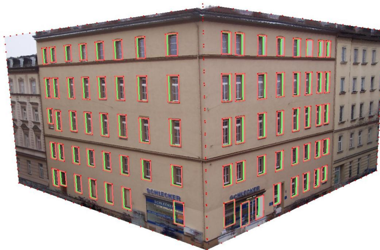
Figure 12: Result for sequence Bordeaux-3 with individual windows constructed from eleven images – explanation cf. Figure 10
