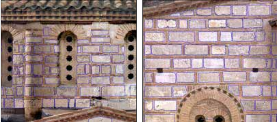
Figure 5. Samples used for the evaluation of the results of the proposed method. Left, part of the drum that supports the dome. Right, part of the stonework of the middle-leveled area of the façade
