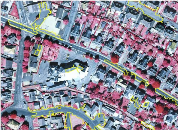
Figure 5. Road parts extracted in subset 3 (yellow).
